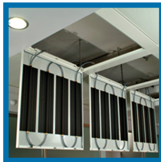
Ceiling radiant cooling panels.
