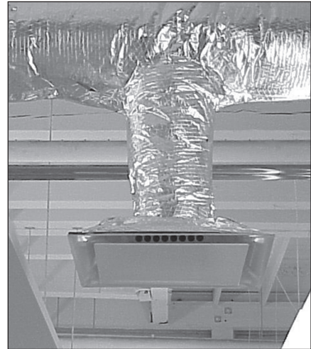
A two-way, high-induction diffuser.
